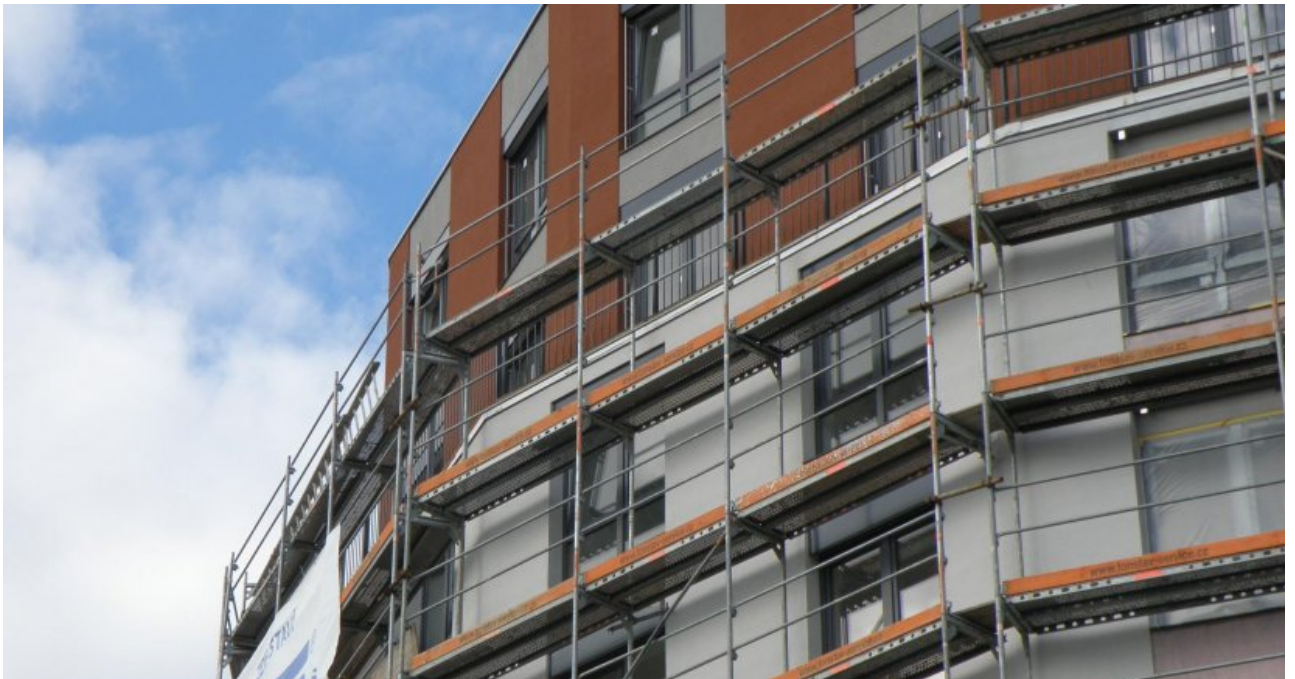
External isolation in a building © Pixabay
